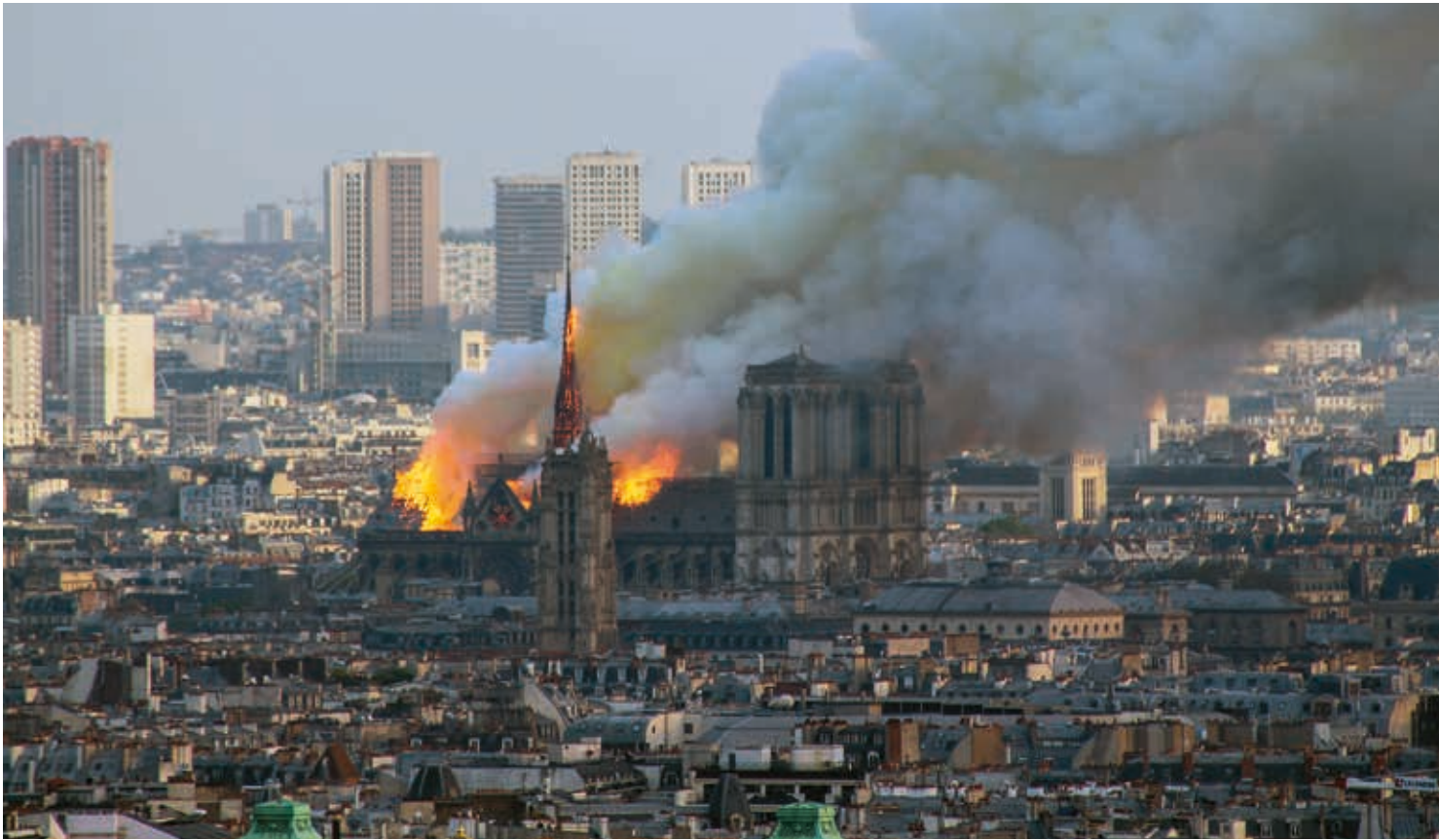
▲ The 2019 Notre Dame Cathedral Fire was caused by an electric fault.
